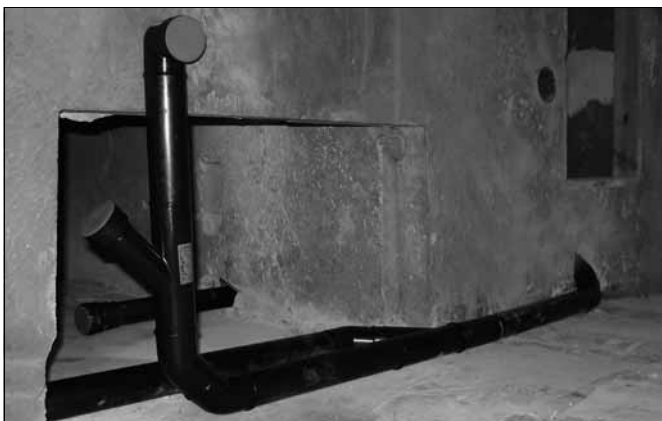
Illustration 6.2 Prefabricated pipe sections installed on site
